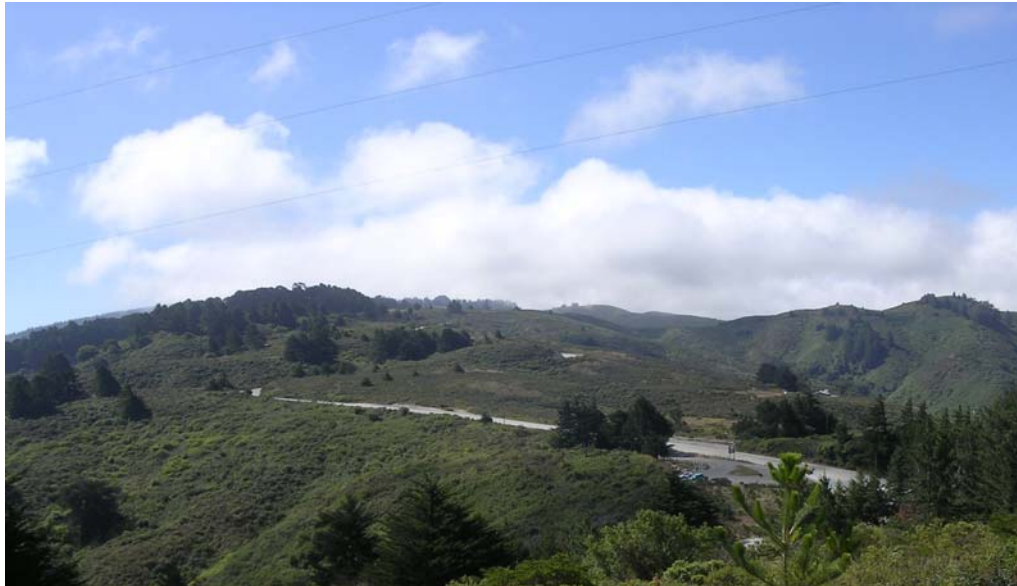
SEGMENT I: VIEW SOUTH FROM ABOVE HIGHWAY 92. CALTRANS PARKING LOT VISIBLE IN LOWER RIGHT.
